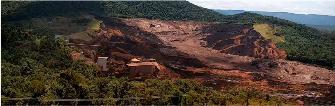
Figure 12: Final Regression of the Failure 6 min and 25 s After the First Observed Deformation, as Captured by CAM1
