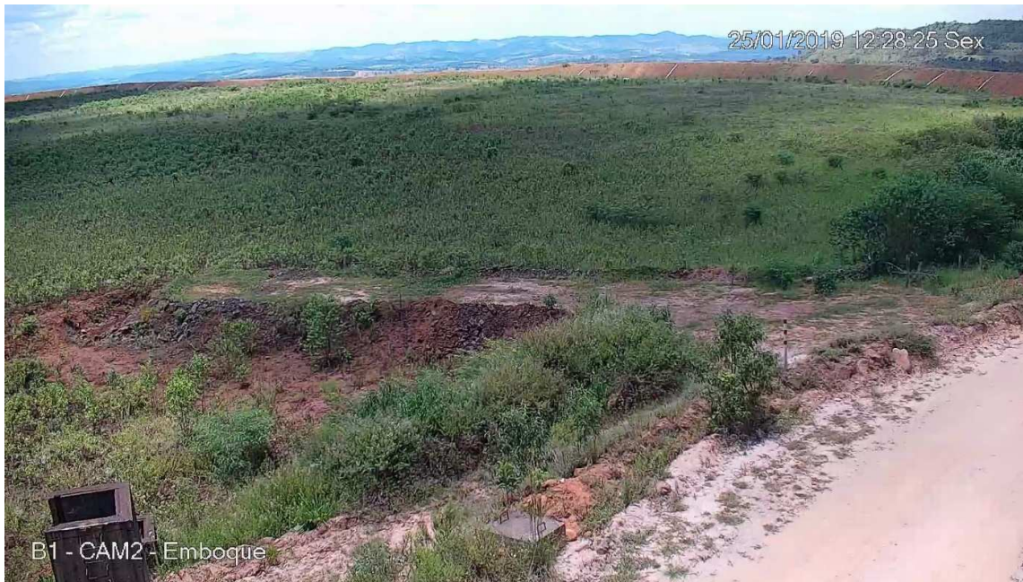
Figure 14: Initial Settlement of the Central Part of Crest, as Captured by CAM2
