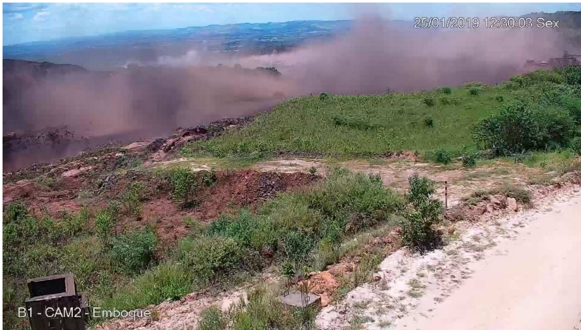
Figure 16: Regression of Liquefaction Failure at 98 s After the First Observed Deformation at the Crest, as Captured by CAM2
