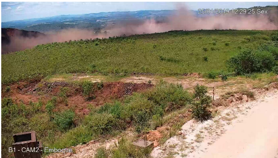
Figure 15: Regression of Liquefaction Failure at 60 s After the First Observed Deformation, as Captured by CAM2
