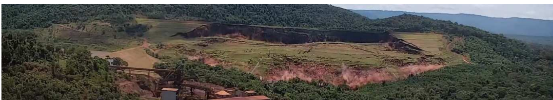
Figure 9: Full Development of Slope Failure with Failed Mass Moving out Beyond the Toe at About 6.7 s After the First Observed Deformation at Crest
