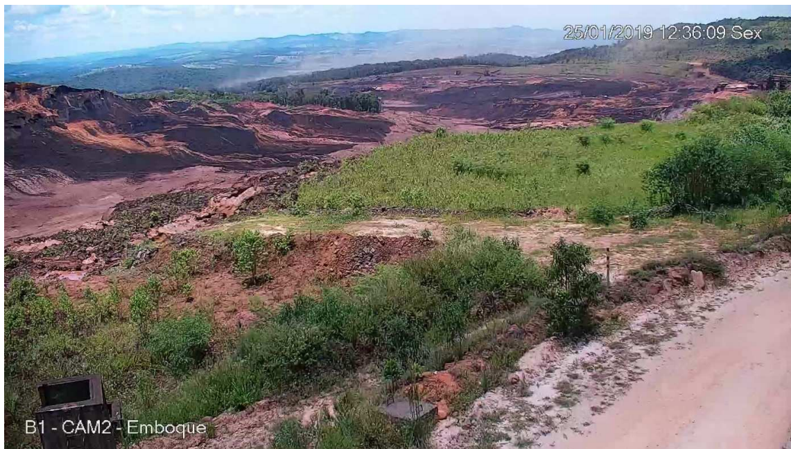
Figure 17: Final Regression of Liquefaction Failure 7 min and 44 s After the First Observed Deformation Initiation of Failure, as Captured by CAM2
