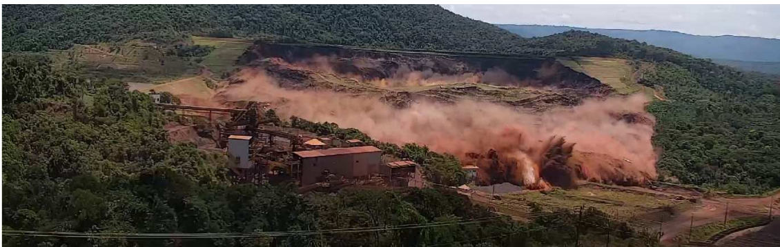
Figure 11: Regression of the Failure 18 s After the First Observed Deformation, as Captured by CAM1
