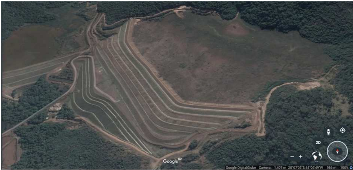
Figure 4: Dam I Looking North (Source: Google Earth 3D, Image Dated July 7, 2018)
