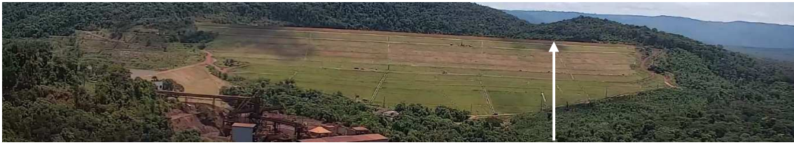
Figure 5: Observed Initial Deformation of the Central Part of Crest
