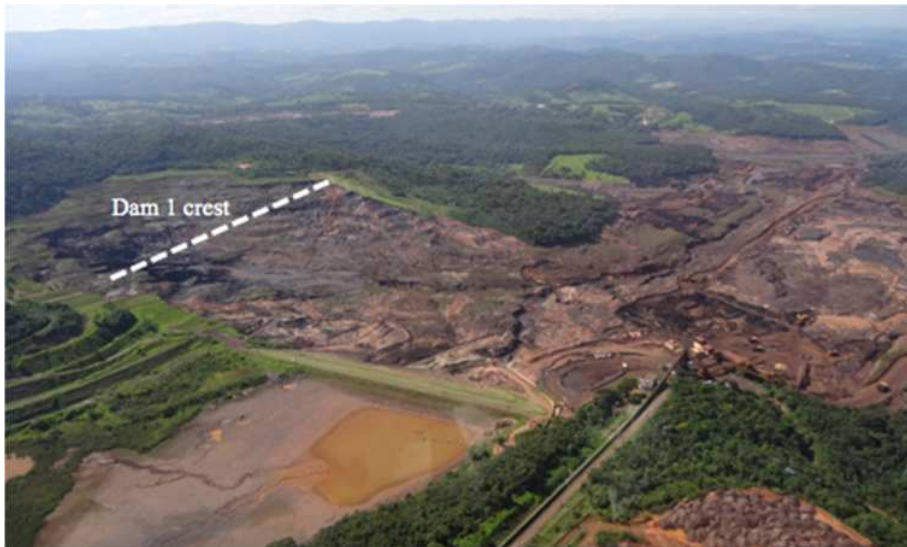
Figure 25: Aerial View of Failed Dam I, Looking Approximately South-East, Photographed on March 28, 2019
