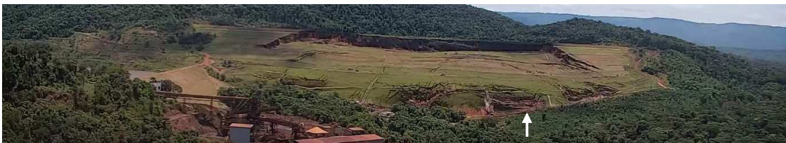
Figure 8: Extensive Settlement of the Crest and Bulging Above Toe with a Second Water Spout in the Region of Bulge About 5.8 s After the First Observed Deformation at Crest
