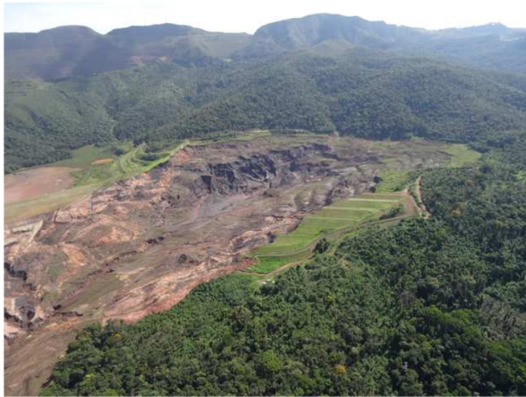
Figure 26: Aerial View of Failed Dam I, Looking North, Photographed on March 28, 2019
