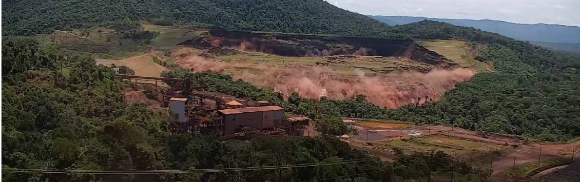
Figure 10: Regression of the Failure 11 s After the First Observed Deformation, as Captured by CAM1
