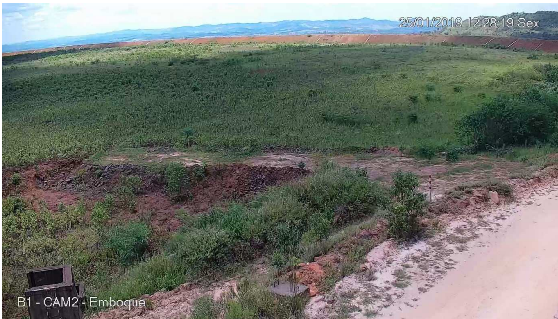
Figure 13: Just Prior to the First Observed Deformation, as Captured by CAM2
